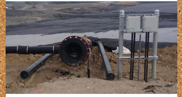
EPG will almost always recommend the use of breakout junction boxes. It's the most economical approach to extending the life of expensive controls. If the decision is made to forgo the purchase and installation of breakout junction boxes, here is a list of conditions that you may be choosing to accept and live with:
