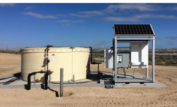
array, and a DC to AC power inverter. The solar panel/battery system provides enough power to operate pump and controls to transfer leachate from the landfill sump/riser to an adjacent storage tank. The control panel is also equipped with a connection for generator provided power as backup.
