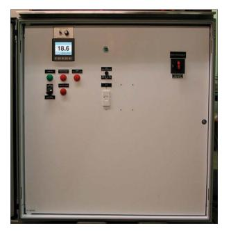
Features include level start/stop set points, high and low level set points (for alarm), high-high and low-low preset points as fail-safe pump shut-off and flow rate and total. Operator friendly screens are easily accessible for display of runtime, number of starts, and alarms. Utilizes a transflective touch screen display that is visible in both direct sunlight and low light conditions.
